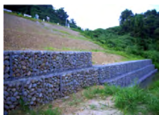
< 盛土のり尻補強 >
